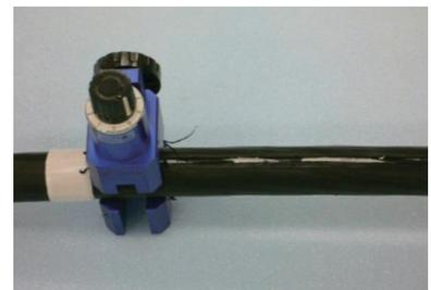
**STEP 4 :** Cut around the cable at the both ends (Circular)
